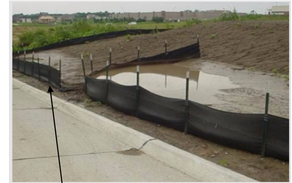
Example of Silt fencing in use Bowman Construction Supply (2023) Available at: < https://www.bowmanconstructionsupply.com/products/silt-fence/ >
