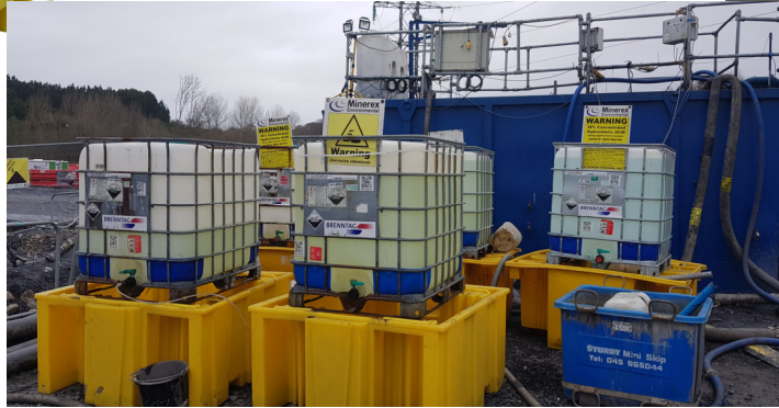
Example of a temporary spill pallet bund (Road Ware, 2023)
