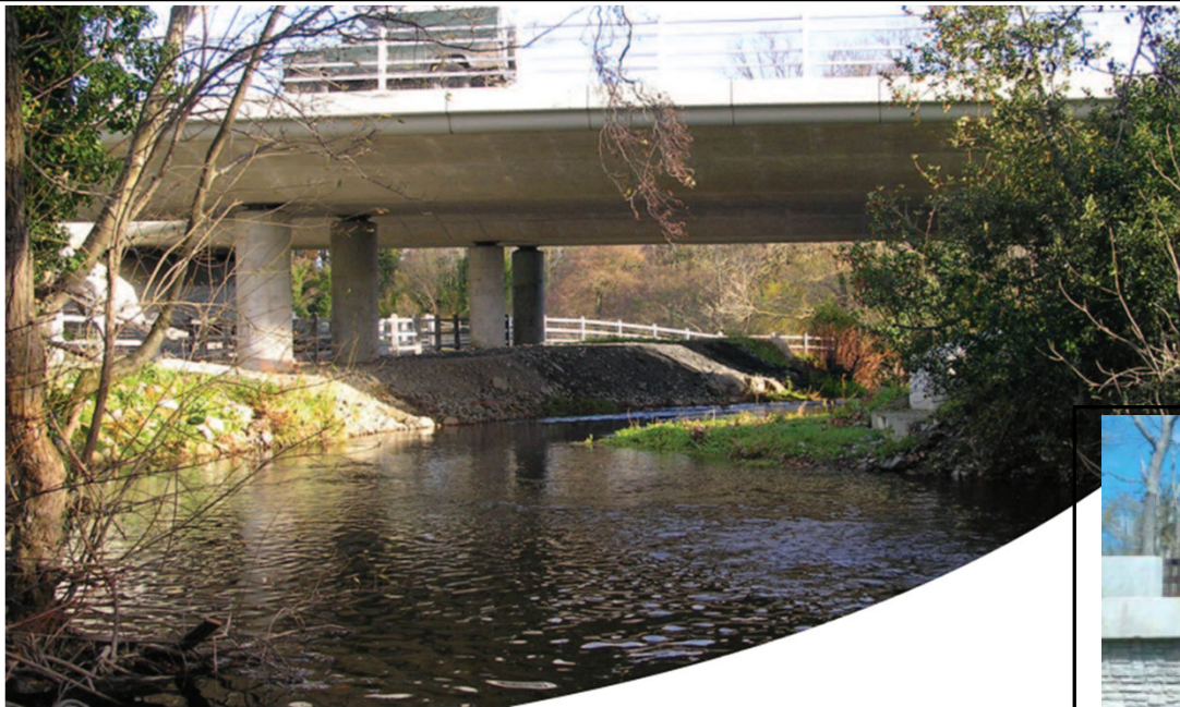
Example of a clear-span bridge, which retains the existing river channel and column set back from the river bank (National Roads Authority, 2008)
