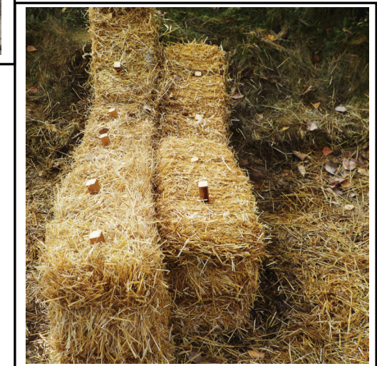
Example of a Strawbale Checked Dam (Kawartha Conservation, 2020)
