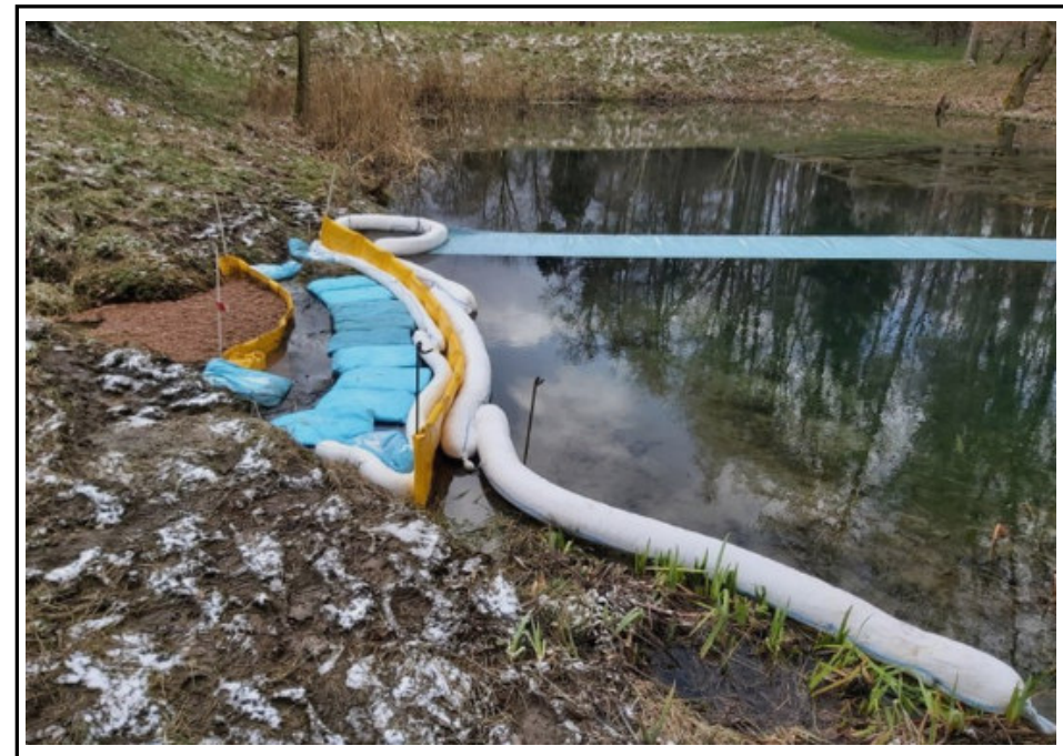
Example of a spill kit deployed in surface water (Oracle Environmental Experts Ltd., 2022) Available at: https://www.oracle-environmental.com/spill-kits
