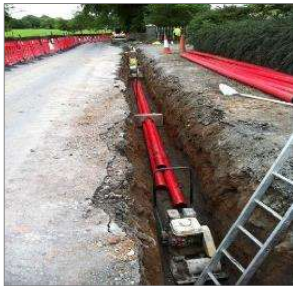
Figure 2 - Typical 38kV Underground Duct Installation
