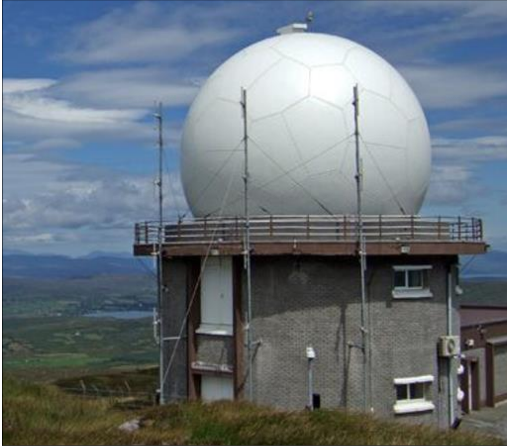
Figure 9. Mt Gabriel Radar Station.
