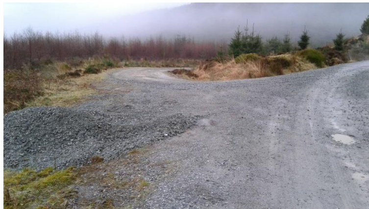
Photo 15.3 – Existing Forest Road at Chainage 1000 m
