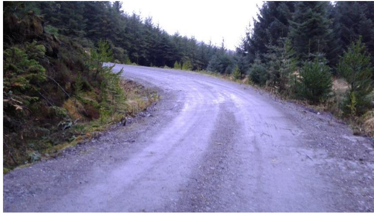
Photo No. 15.4 – Existing Forest Road at Chainage 1800 m
